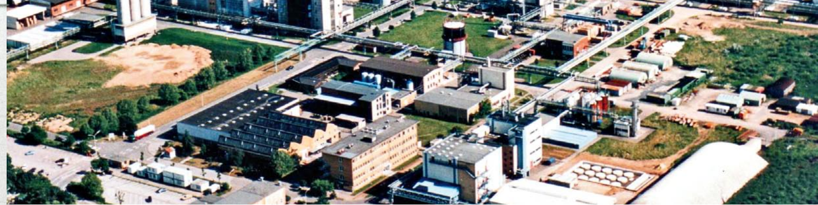
Wacker Chemie has relied on PROFIBUS PA at its Cologne facility since the 1990s
