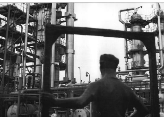
Schwedt oil refinery paraffin unit in 1972. Over 30 years later, a unit based on PROFIBUS PA was built here by the Verbio Group, a leading manufacturer of biofuels and the only large-scale industrial producer of biodiesel and bioethanol in Europe
