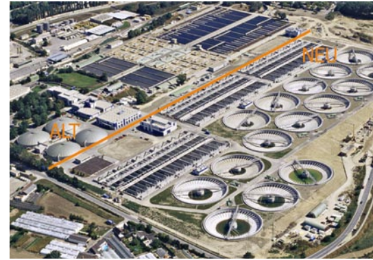
The wastewater treatment plant in Vienna relies on PROFIBUS PA – and is one of the most modern facilities of its type in the world.
