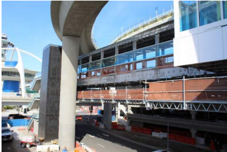
Figure 1 – ECTA Viewing Pavilion
